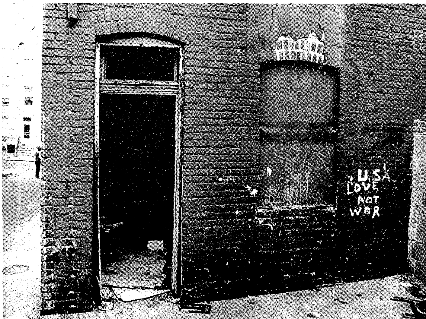
Lubec Town hall looks ready to be demolished under new disaster bill.
