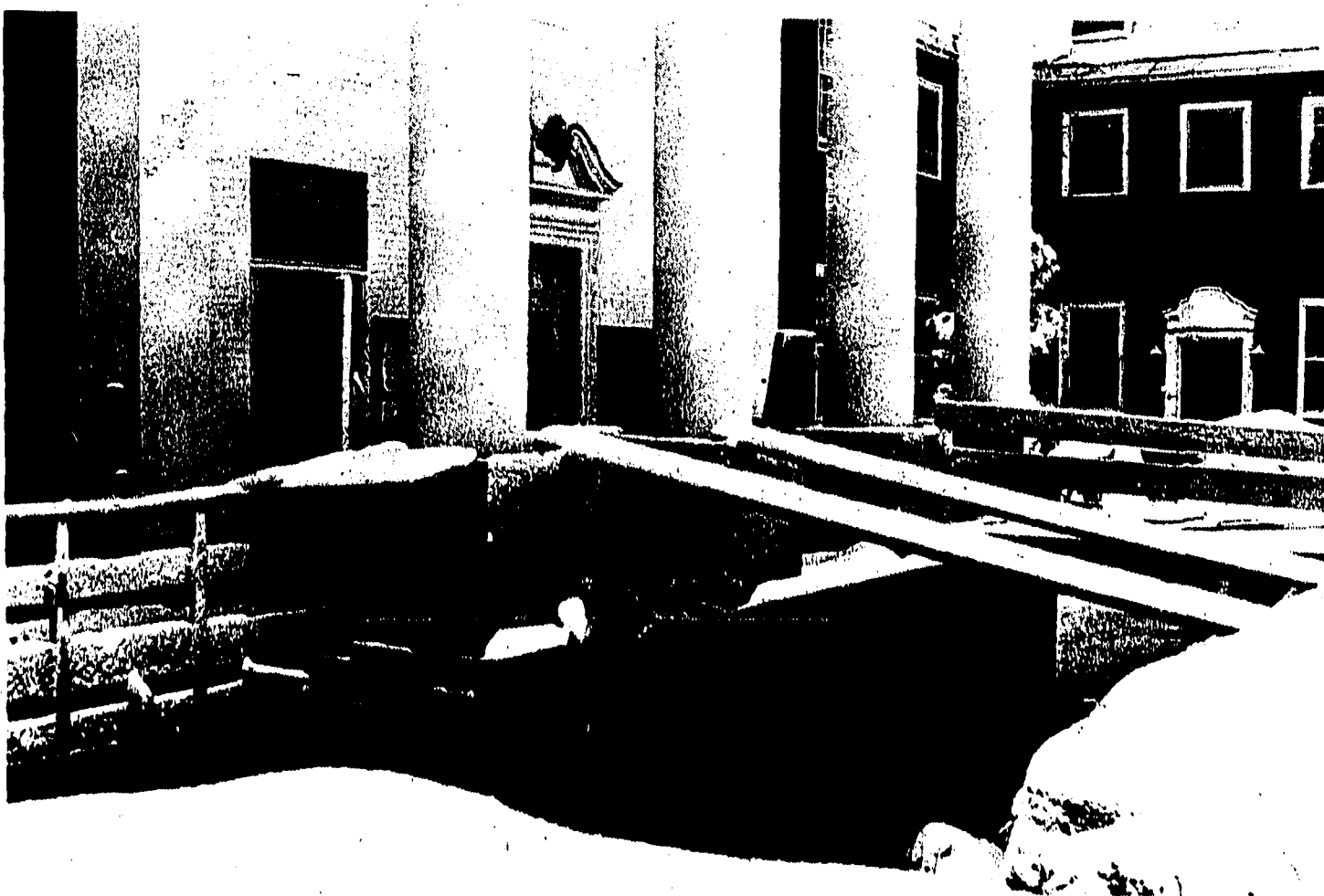
Roberts renovation is underway (Photo by Richard Highland)
