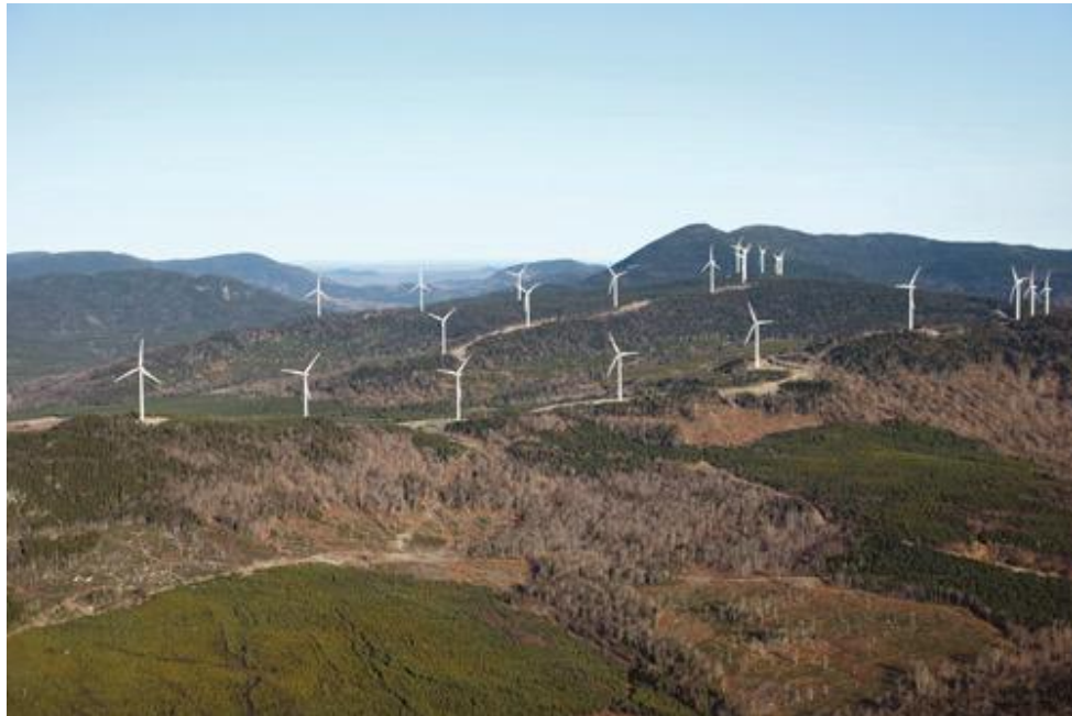
Image 1: Kibby Wind Farm is a 44-turbine farm located on Kibby Mountain in the Boundary Mountain Range near Eustis, Maine. Construction on the project began in 2007, and the turbines began to spin in 2010. The main concerns with Kibby are the habitat destruction and destruction of the mountain range's beauty.
