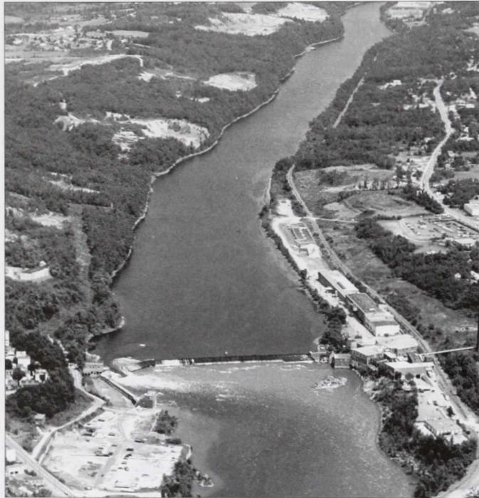
On July 1, water smashes through a breach (at left) in Edwards Dam on the Kennebec River, setting a national precedent for river restoration.
