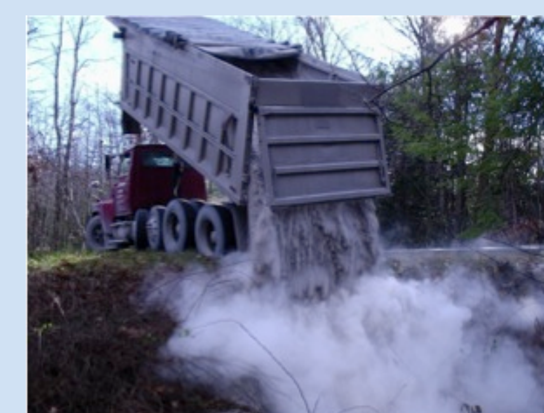
Limestone sand dumped into a stream affected by AMD 2
