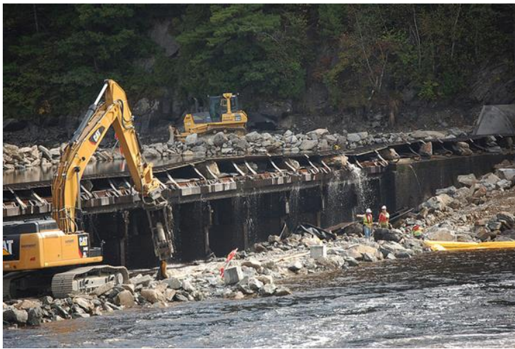
Figure 3. Removal of the Veazie Dam (2013).
