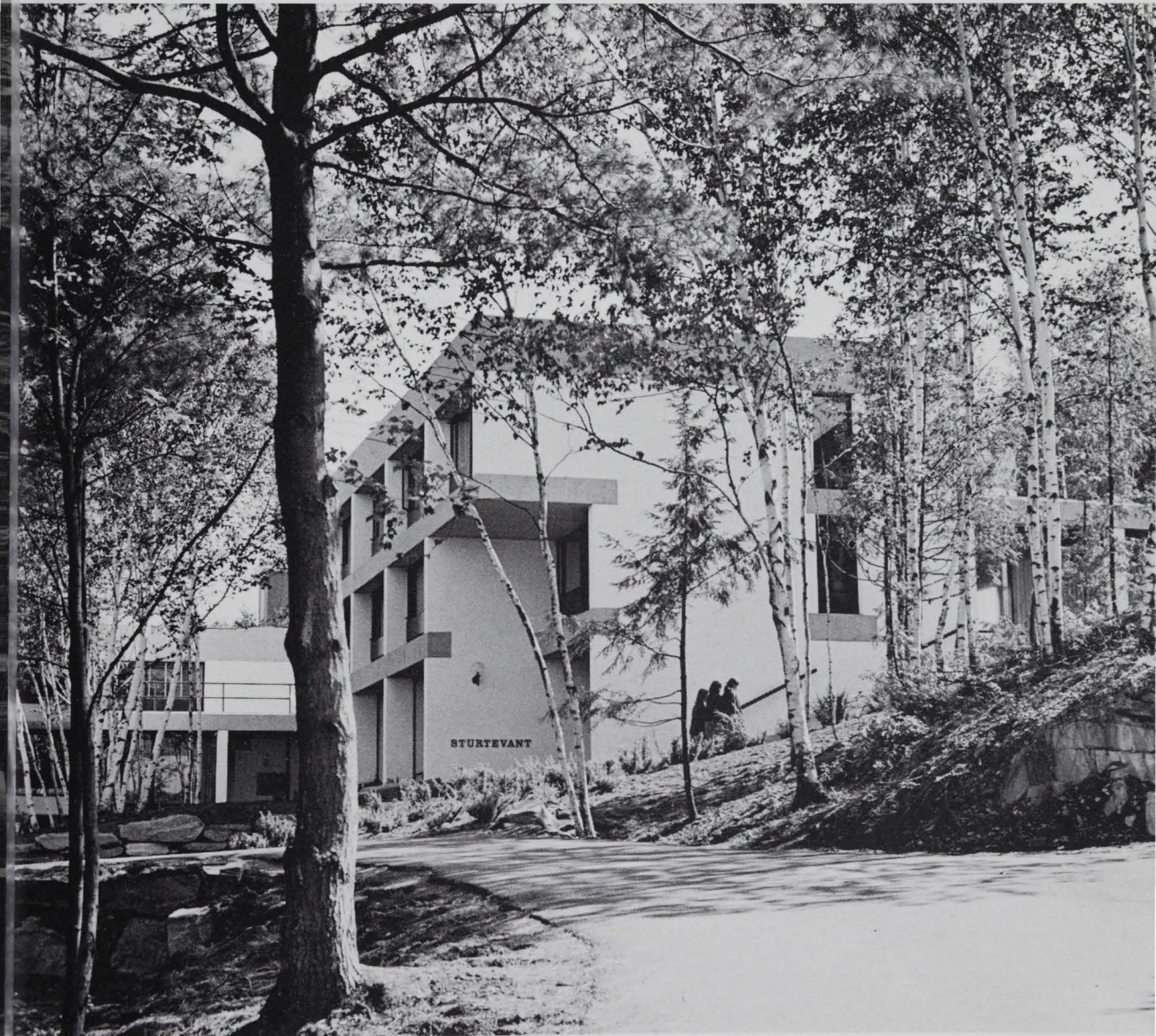
Award-winning dormitory complex
