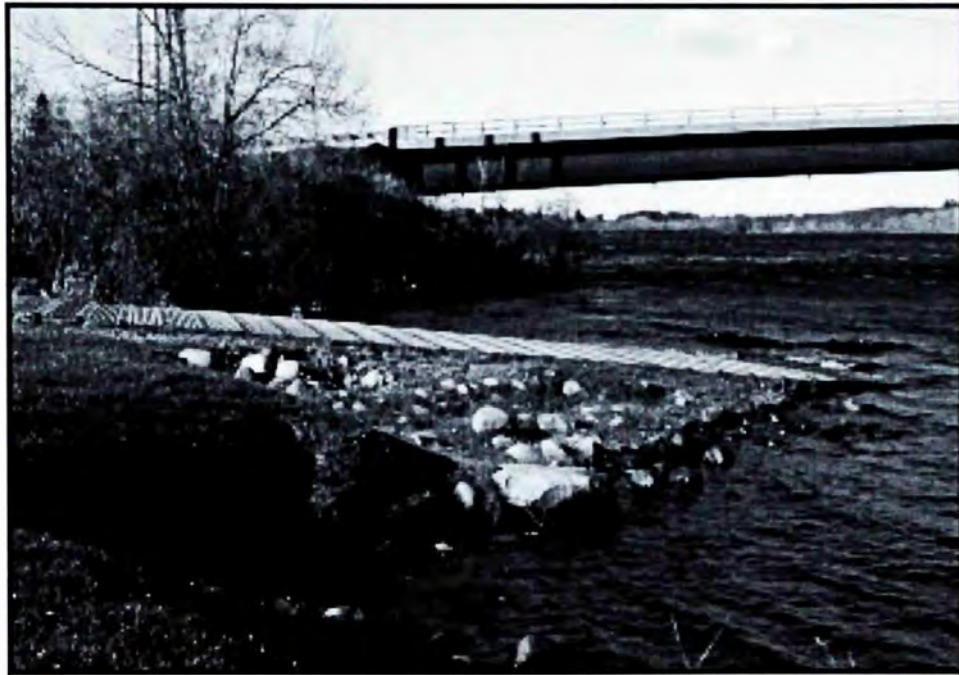
Figure 58. Hinckley boat launch located on the Kennebec River. This launch is more ecologically friendly than the Lake George public boat launch because it is narrow, more buffered, and made of concrete.
