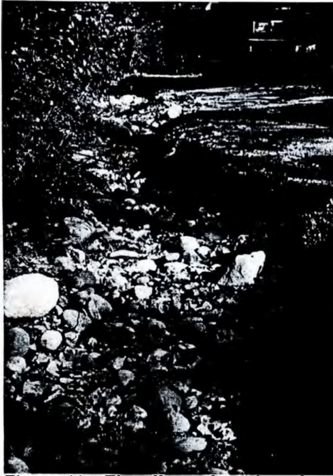
Figure 44. The effects of erosion where a ditch has not been properly maintained.
