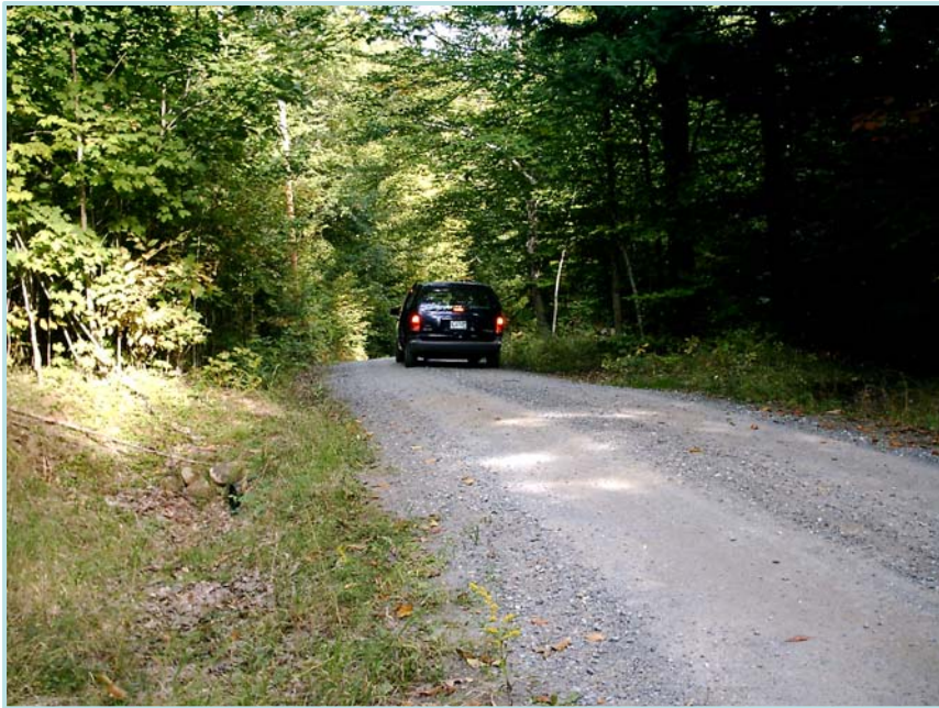
Crowning, grading, and ditching
