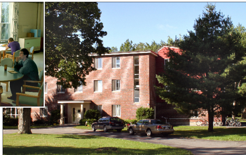
Colby Gardens, a former home for the Ursuline Sisters, is a temporary dormitory. The residence, located a half mile from the main campus, has a fitness center, spacious lounges, and a dining area, shown at left.
