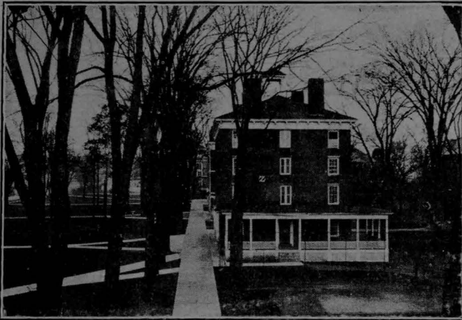
VIEW OF CAMPUS FROM LIBRARY WINDOWS Showing New Granolithic Walks
